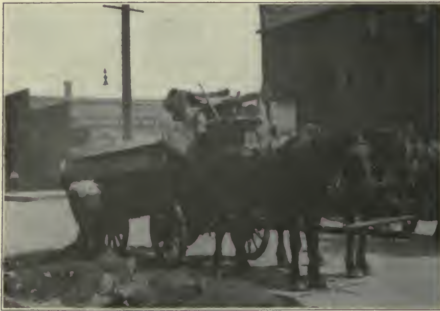
FIG. 61. STREET CLEANING OPERATIONS, A SOURCE OF DUST. In the common method of cleaning streets in Chicago, the refuse is swept into piles in the gutter to be collected later by teams. During the process of loading the wagons, the wind has full opportunity to blow out the finer particles. The gutter is left but "shovel clean" and these leavings in time add to the dust content of the atmosphere.
